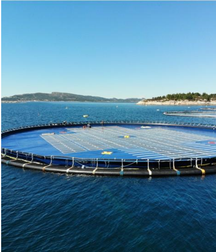
Floating Solar Energy Converters
